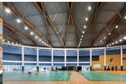
The 48.4-metre cable-stayed dome at the Chengdu Tianfu Fitness Centre.
