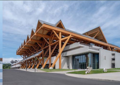
The Shenzhen Guangming International Equestrian Centre, with its 96-metre glulam roof.
