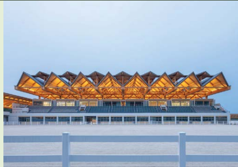
The Shenzhen Guangming International Equestrian Centre, with its 96-metre glulam roof.
