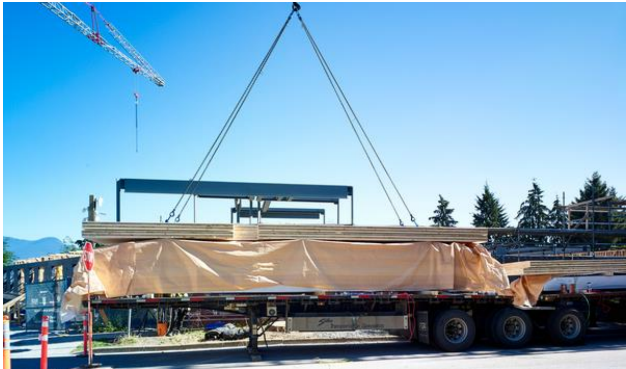
Panel delivery for Vienna House, Vancouver | Credit: Wade Comer Photography
