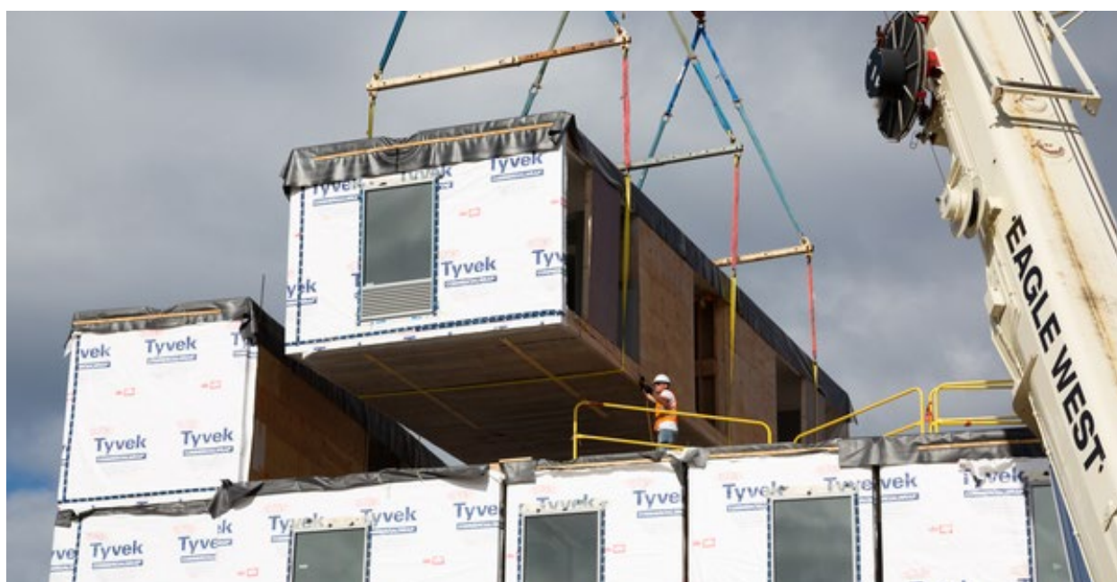
Modular housing construction—Kelowna Airport Hilton Hampton Inn, Kelowna, B.C. Photo credit: Jason Babakaiff Photography, courtesy Blackbox Offsite Solutions
