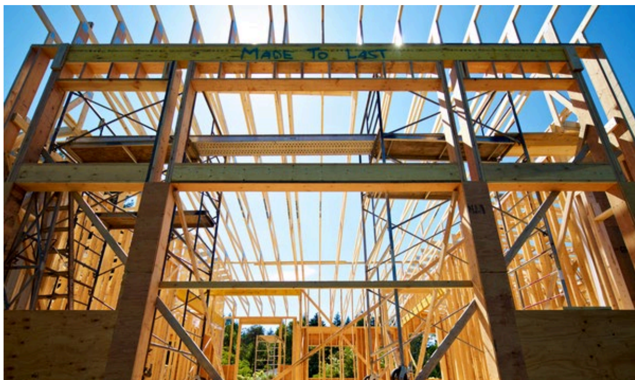
Light wood house frame, Vancouver Island, B.C. | Photo credit: Nik West
