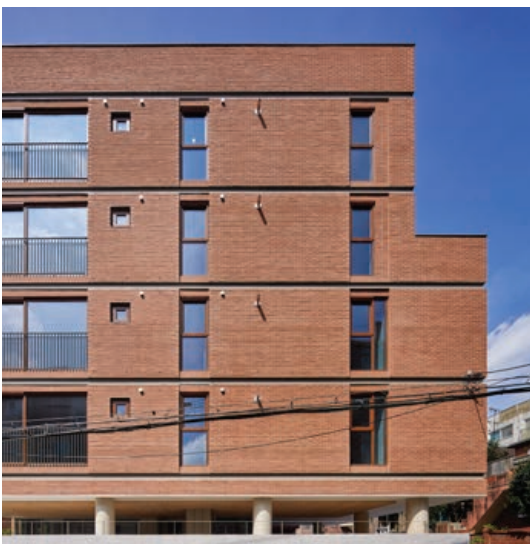
A midrise project in Korea that applies the Wood Infill Wall system using Canadian S-P-F | Photo: Canada Wood
