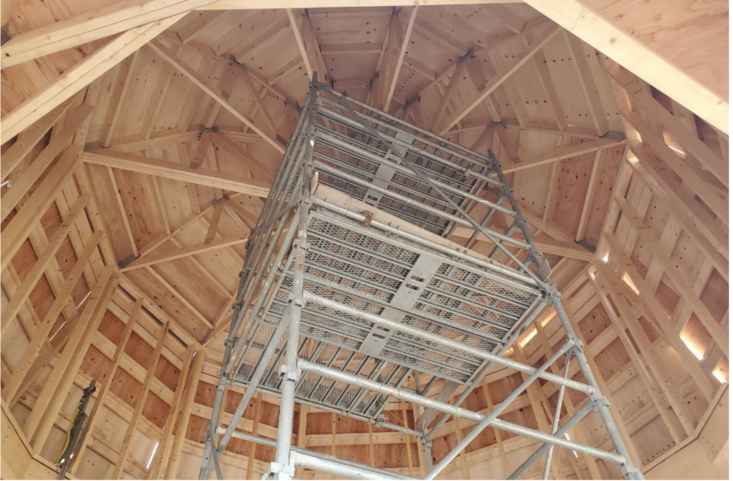
Yuyukai Social Welfare Corporation's nursing home project, Takamatsu | Photo: Canada Wood Japan
