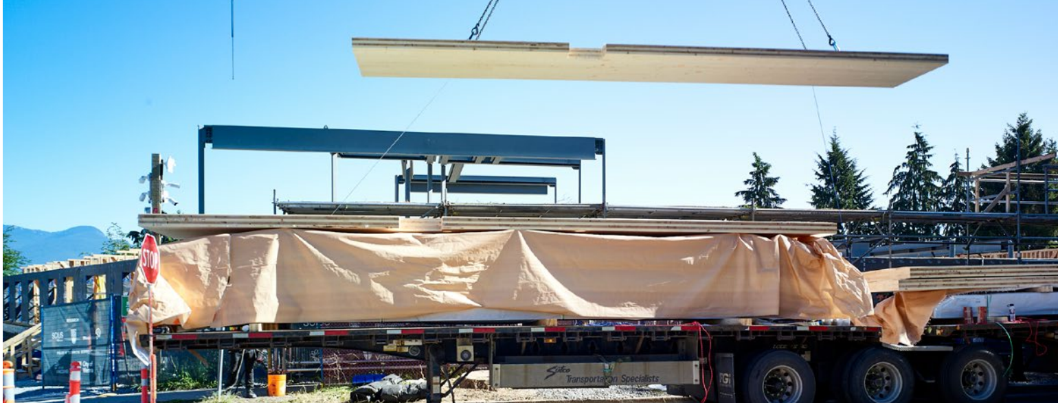
CLT panel lift for Vienna House construction | Photo credit: Wade Comer
