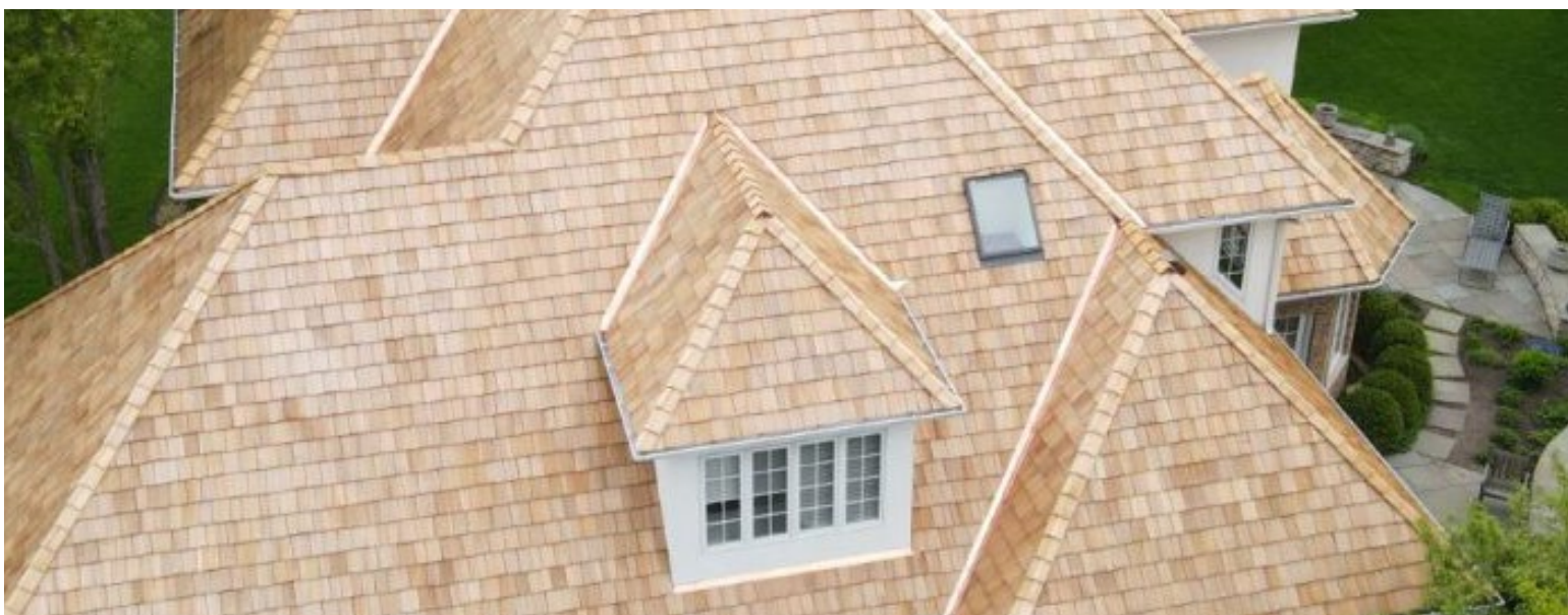
Western red cedar shake shingle roof, U.S. Photo credit: Cedar Shake and Shingle Bureau
