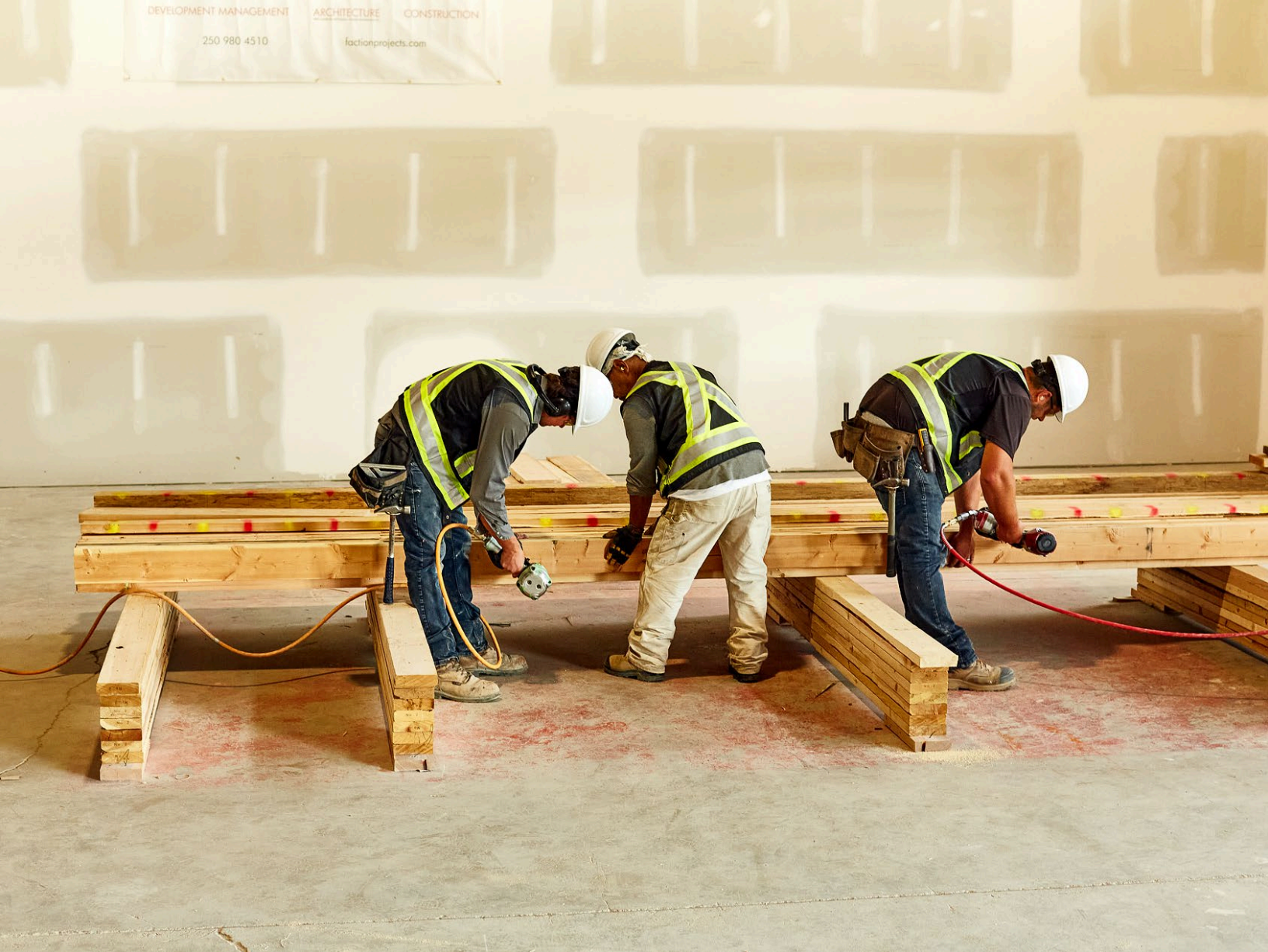
Fabrication process of four NLT panels | Credit: Wade Comer Photography
