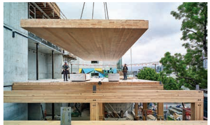
Construction of Man6 - CLT panel placement | Photo: Wade Comer Photography, courtesy naturallywood.com
