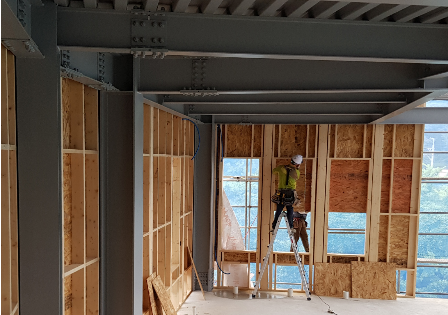
Cheongpyeong Cultural Centre steel and wood infill wall project, Gyeonggi province | Photo: Canada Wood Korea
