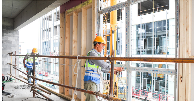
C-Mars Office Project—installing the prefabricated wood wall | Photo: Canada Wood China
