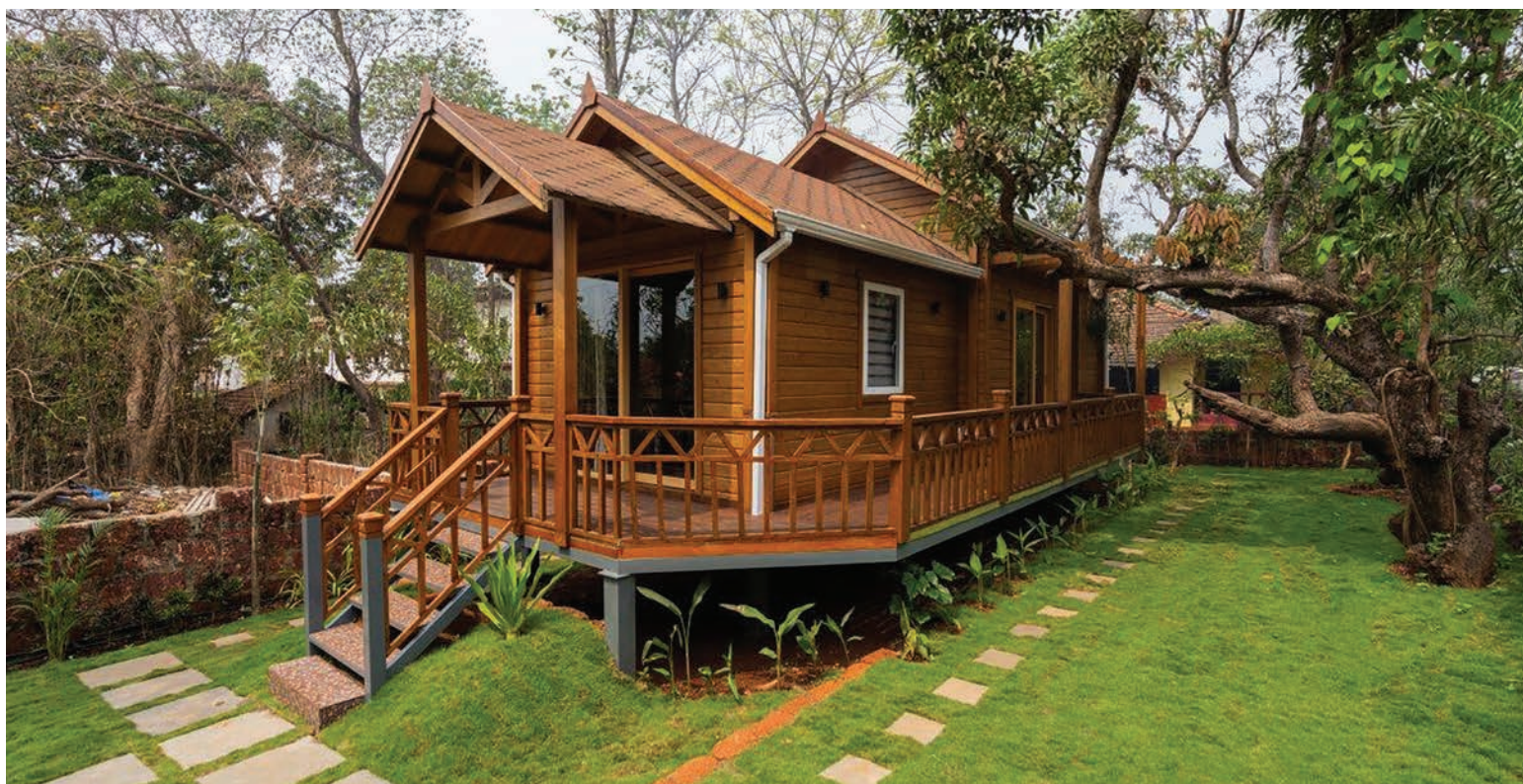
Laminated tongue & groove resort-style cottage built by Woodbarn India, now on display in Goa.
