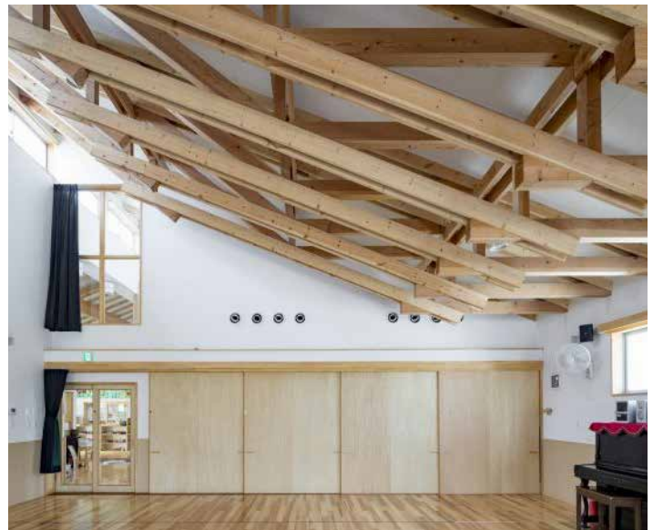
The one-story Ozeki nursery school has a total floor area of 998.25 m 2 , and uses dimension lumber for rafters and trusses.
