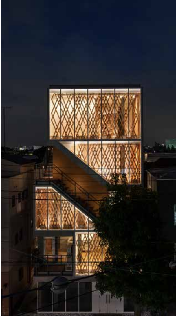
The second 2x4 wood-framed five-storey building to be built in Japan, and the first in central Tokyo. Shimouma Apartment is an 18 metre tall building that contains a cafe on the first floor, rental apartments with nursing services for aged patients on floors two and three, and staff rooms on floors four and five.
