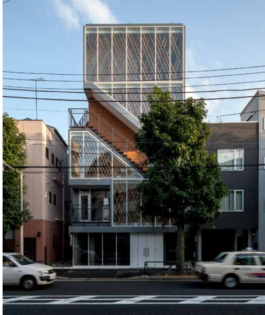
The second 2x4 wood-framed five-storey building to be built in Japan, and the first in central Tokyo. Shimouma Apartment is an 18 metre tall building that contains a cafe on the first floor, rental apartments with nursing services for aged patients on floors two and three, and staff rooms on floors four and five.
