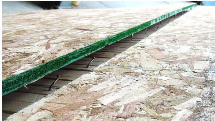
Figure 7 Nail head pull-through and withdrawal failure
