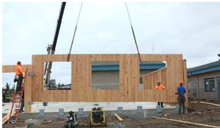
Figure 16. Installation of CLT Wall Panels at Grey Wolf Elementary in Sequim Washington, US
