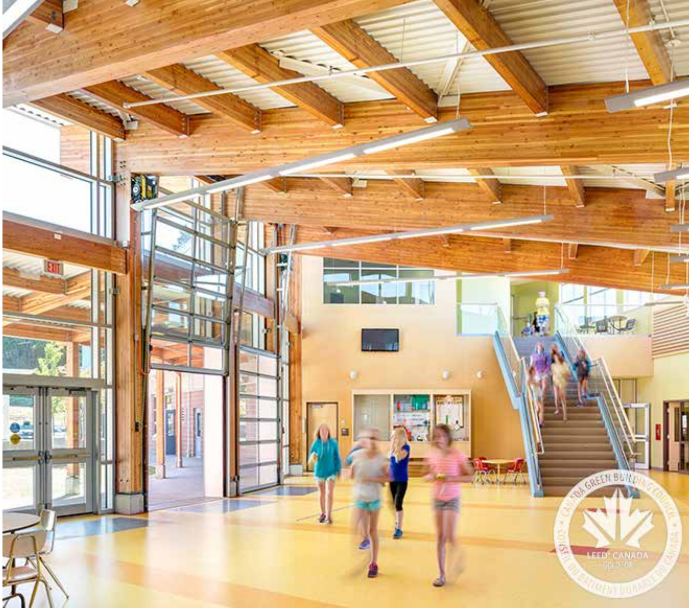
Figure 26. Westview Elementary School (School District 47) Powell River, British Columbia – Post And Beam Construction With Glue Laminated Timber (GLT)
