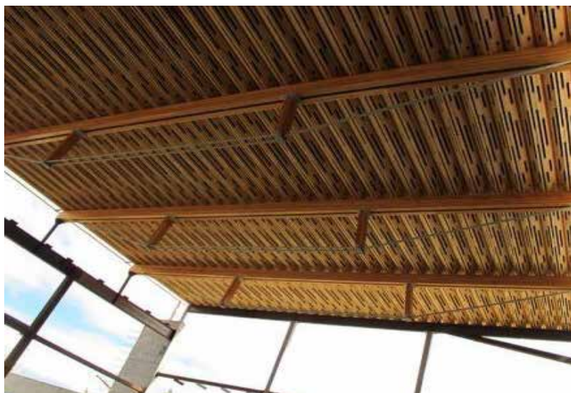
Figure 28. Port Alberni Secondary School (School District 70) Port Alberni, British Columbia—WoodWave Structural Panel System Used to Meet Structural, Architectural, Acoustic, and Sustainability Objectives
