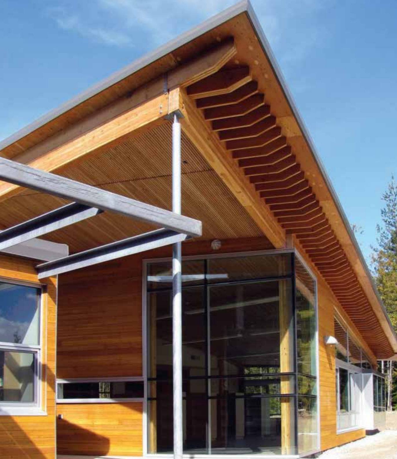
Figure 8. Crawford Bay Elementary–Secondary, School District No. 8—Roof Overhangs Designed To Protect Exposed Wood
