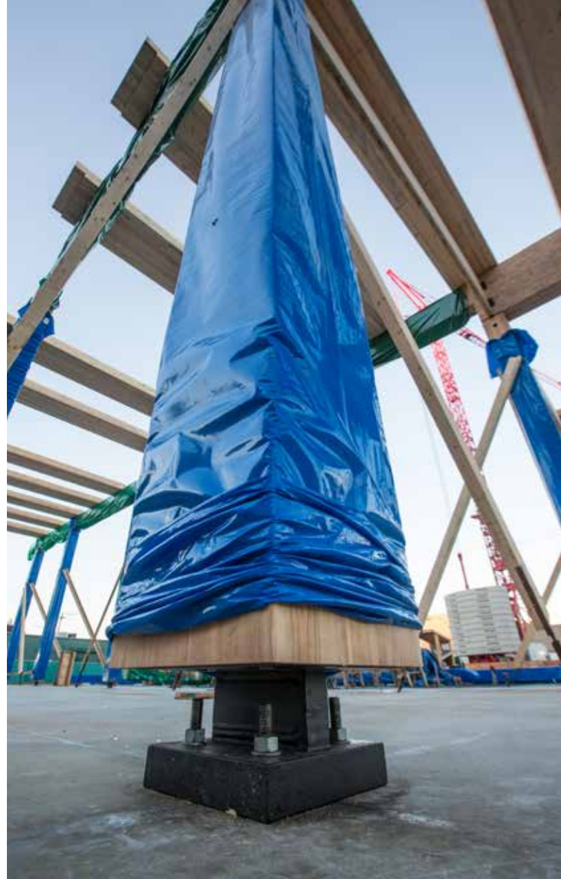
Figure 4. Glulam Columns Protected During Construction of the Wood Innovation and Design Centre in Prince George
