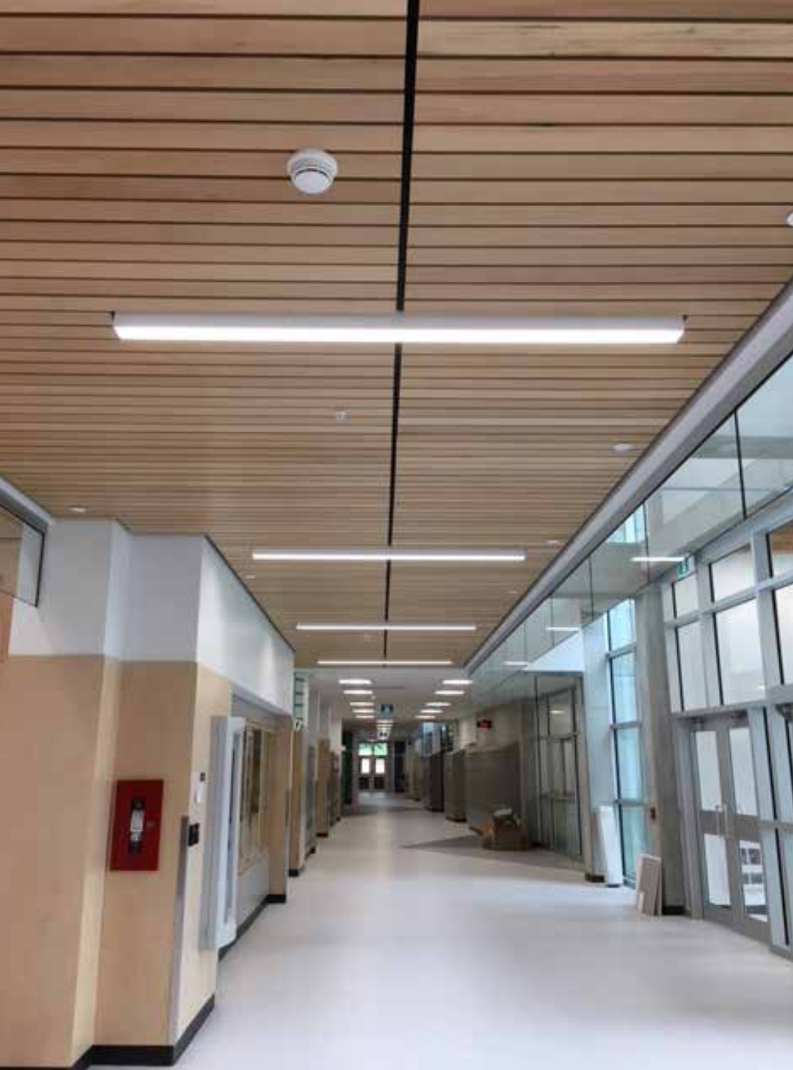
Figure 9. Linear Wood Slats Used on Ceiling for Acoustic Absorption and Aesthetic Finish at Salish Secondary School in Surrey, BC
