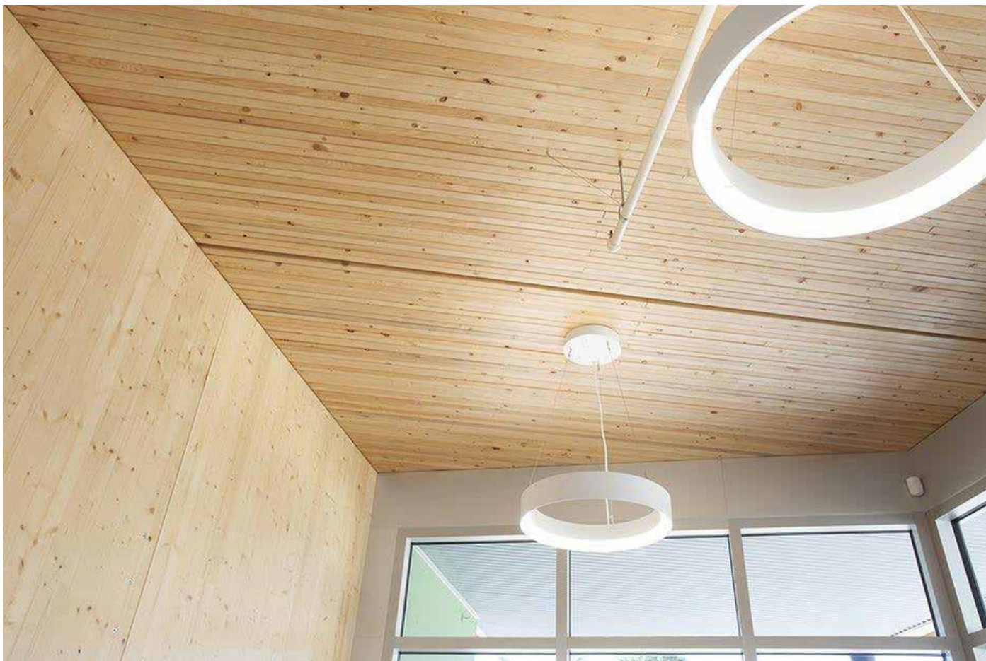
Figure 27. Cordova Bay Elementary School (School District 63) Victoria, British Columbia—Exposed CLT Walls and NLT Roofs
