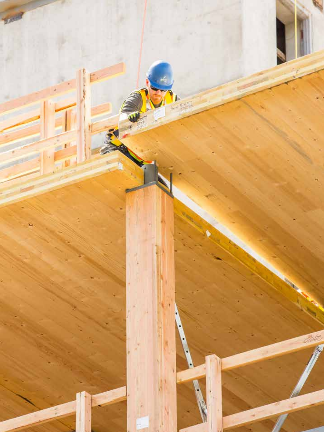
Figure 5. Installation Of Pre-Fabricated Mass Timber Floor Components for Brock Commons Tallwood House at the University of British Columbia
