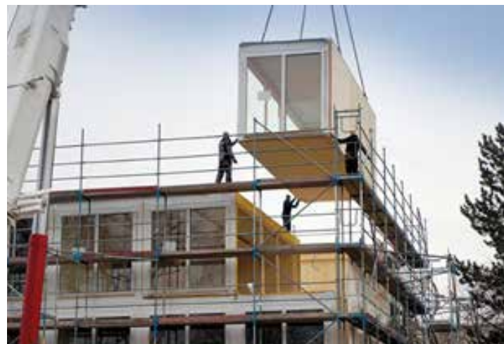
Figure 18. Prefabricated Classroom Module Being Installed On Site, Frankfurt, Germany
