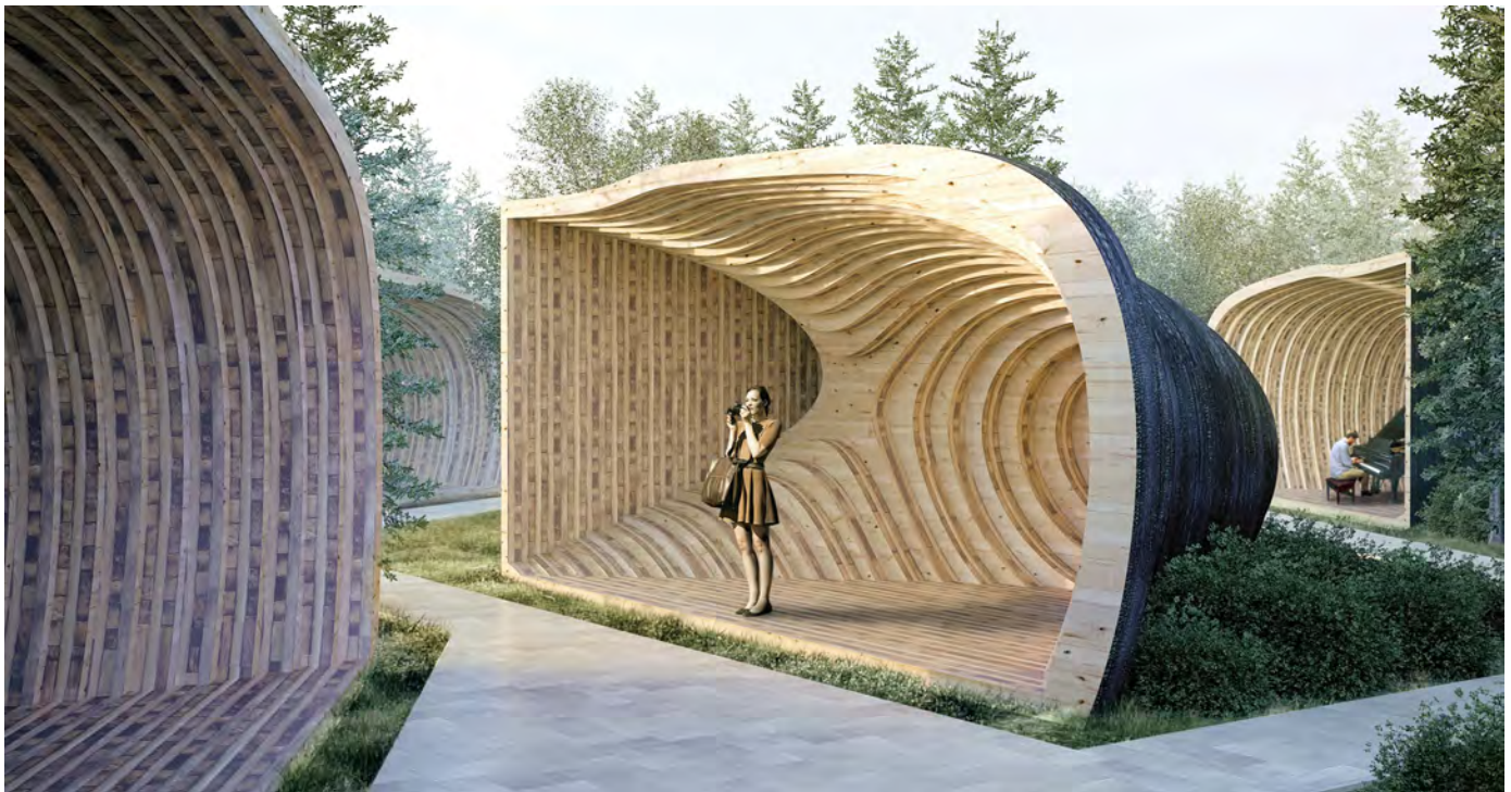
Figure 18. Render of a lapped CLT structure
