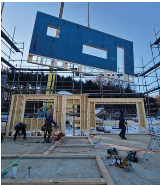
Maple Village Super-E house construction / Photo: Canada Wood Korea
