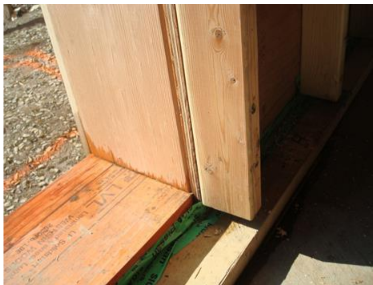
Figure 5 A photo of the double-stud wall of the house
